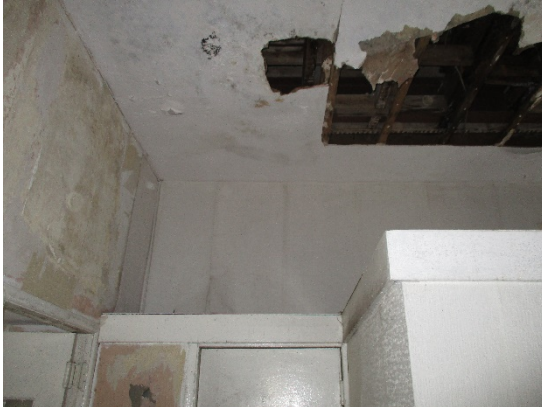
Plate 11: Gaps in attic ceilings
