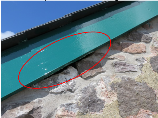
Plate 13: Example of bat access slit at gable wall fascia
