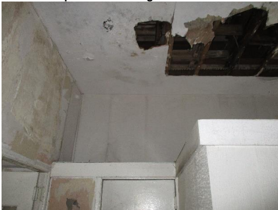
Plate 11: Gaps in attic ceilings
